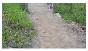
The Rotary Vista Trail was damaged in early 2016 during a January thaw that attracted hikers and resulted in deep footprints in the trail surface. The trail surface was still pockmarked and uneven in late April 2016.
