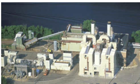
Xcel's WTE facility - French Island
