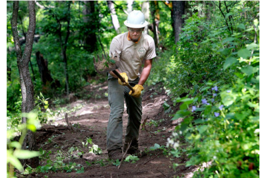
Trail Building at Landfill by Wiscorp
