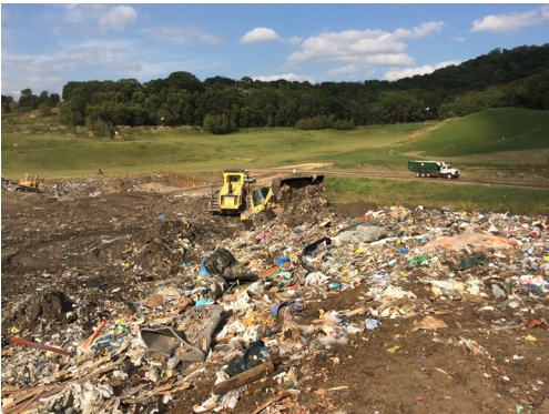
Phase VIII waste placement and compaction
