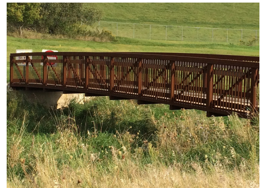
Pedestrian Bridge over wetlands completed by Eagle Scout Brant Attleson
