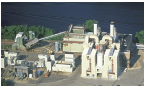
Xcel's WTE facility - French Island
