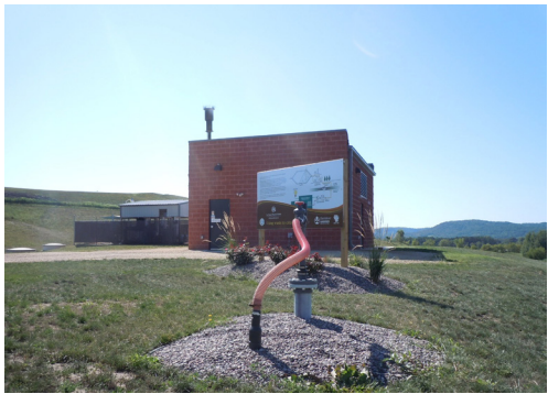
Landfill Gas to Energy Facility
