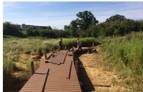
Photo of Boardwalk construction at landfill
