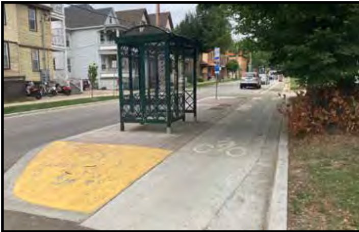
Bus Stop Curb Extension
