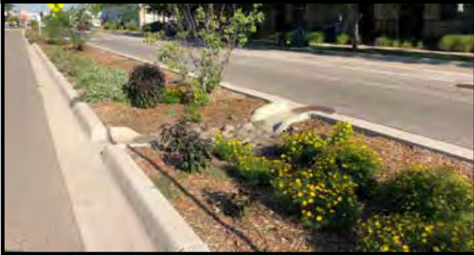
Green Infrastructure for Stormwater
