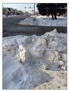
Figure 23: Hardened pile of snow blocking curb ramp and crosswalk at 8<sup>th</sup> St and Cass St.
