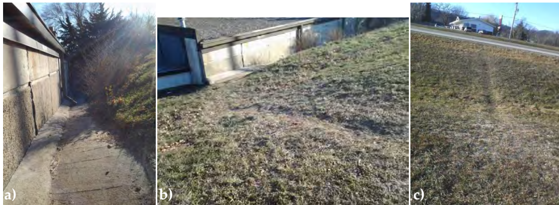
Figure 4-20: Pedestrian path between mobile home park on east side of TH 14/61 to Kwik Trip and other businesses on the west side of the highway in La Crescent, Minnesota.
