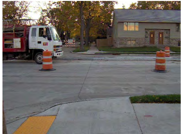
Figure 3-23: A median barrier at West Ave and Mississippi St.
