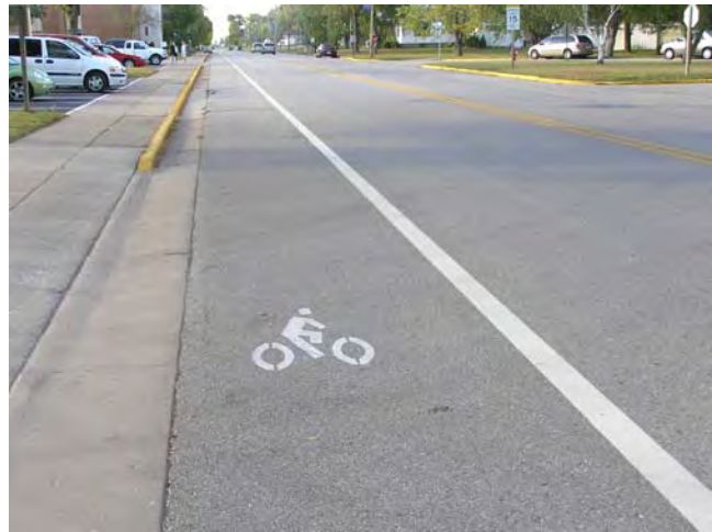
Figure 3-5: A northbound bike lane on the west side of Main St in Holmen.
