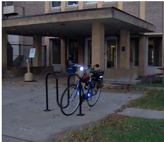
Figure 3-18: An unsheltered 3-loop wave rack. This rack could have been sheltered by the building’s overhang.
