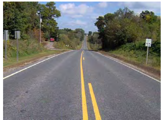
Figure 3-11: Unpaved shoulders of CTH B in the Town of Hamilton.
