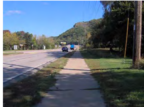
Figure 3-13: The 6-ft sidewalk of the STH 16 Sidepath looking north from La Crosse
