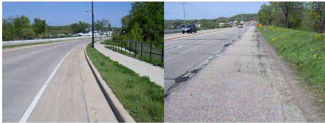
Figure 3-10: Paved shoulders along USH 14/61 between La Crosse and La Crescent. They provide ample space for class A bicyclists. The sidewalk (picture, left), however, is too narrow to accommodate two-way travel of class B/C riders and pedestrians.
