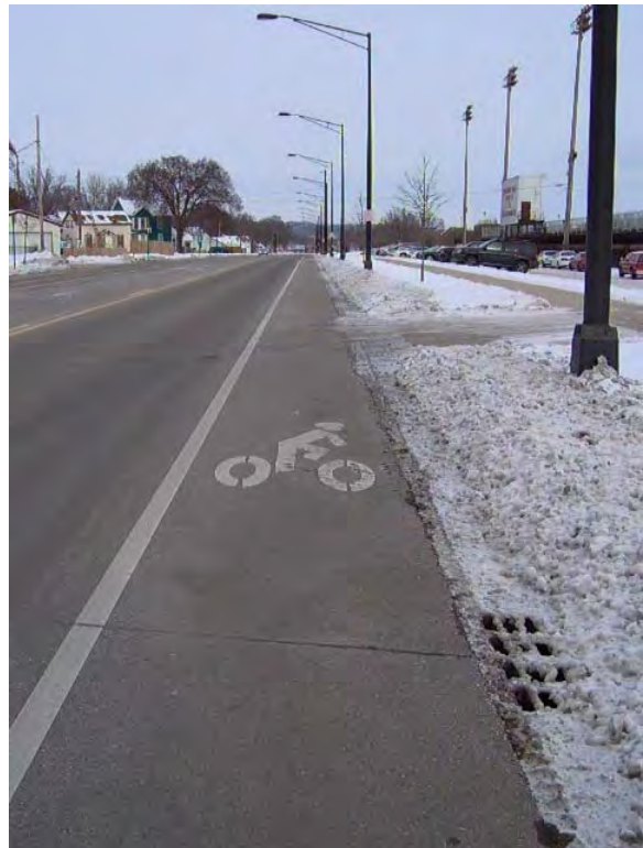
Figure 3-1: Bike lane on Ranger Dr in La Crosse. This bike lane is designated by pavement markings and signage.
