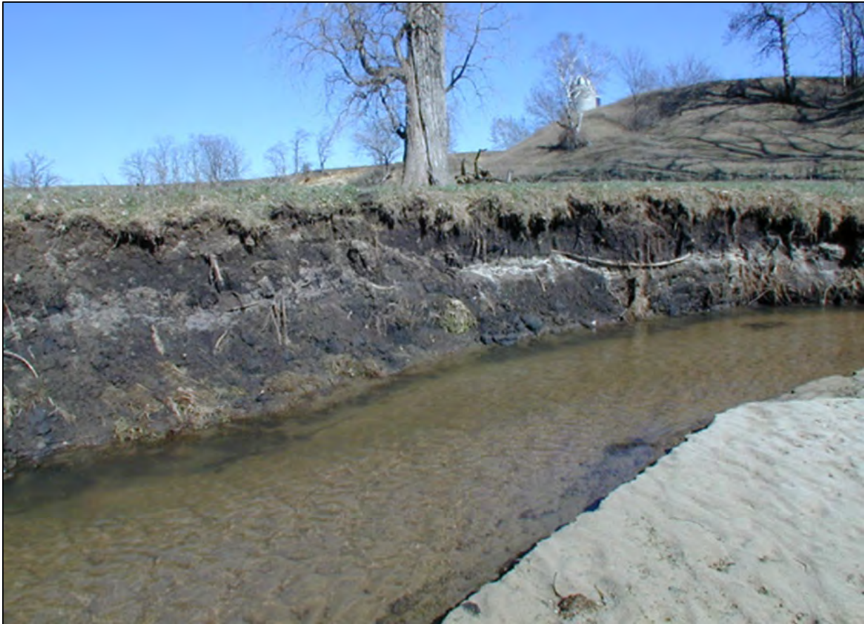
Figure 18 Streambank Erosion Photo
