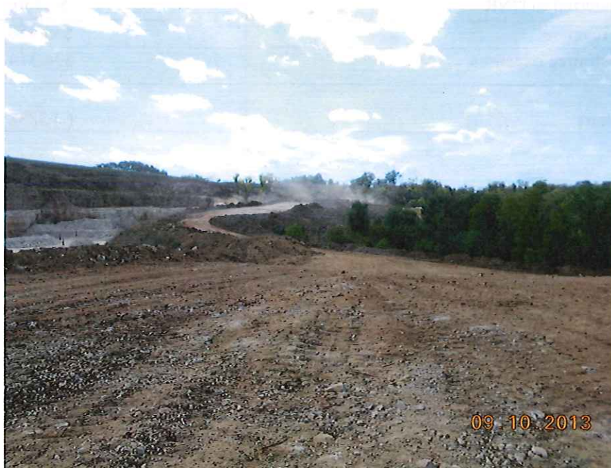
Photo 2 – The Waldenberger Quarry – While on site, Mary Jo addressed an erosion control issue dealing with unstabilized berms and an unprotected slope.
