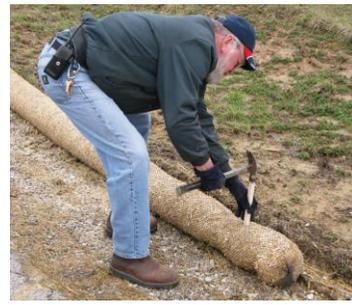
Straw Wattles are an effective and economical alternative to silt fence and straw bales for sediment control and storm water runoff.
